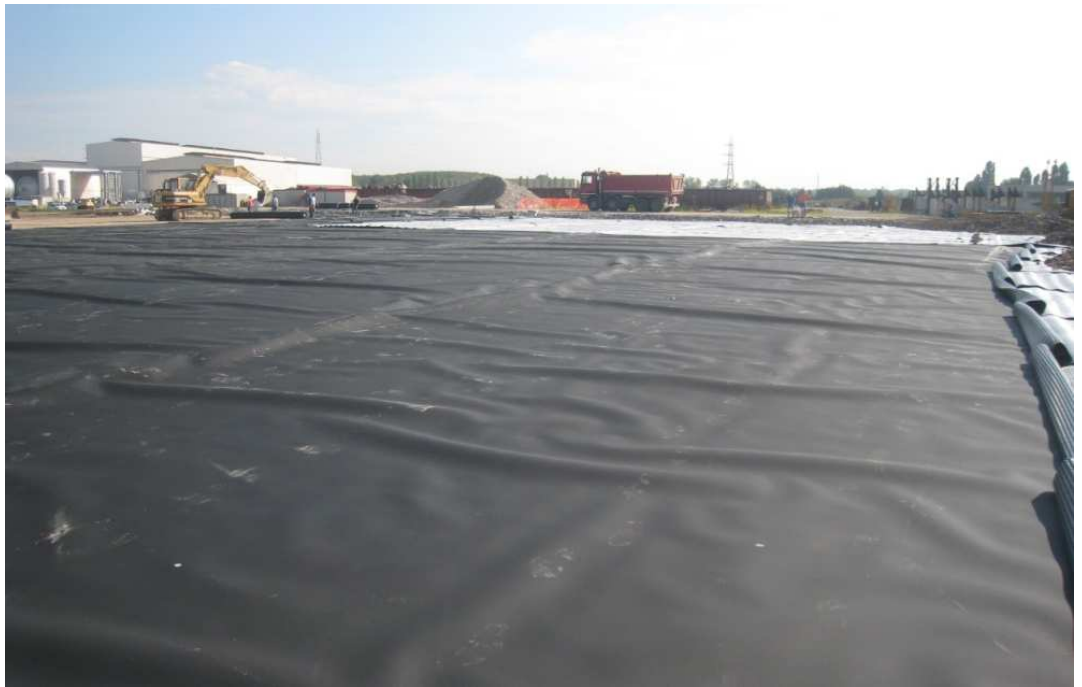
Installation of HDPE smooth membrane in direct contact with contaminated soil;
