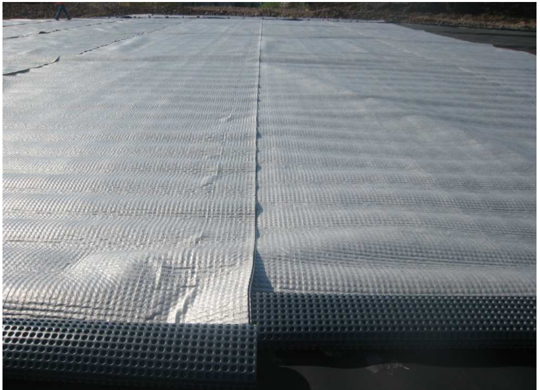
Detail of Isostud Geo P product used above geomembrana in HDPE
